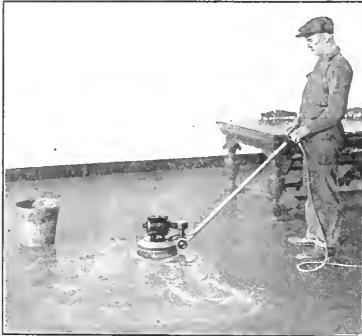
FIG. 3 THE FIRST STEP IN RENEWING AN OLD LINOLEUM FLOOR IS SCRUBBING*
